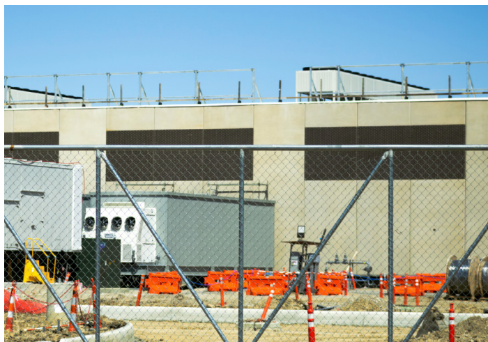
Data center being built in Central Ohio. Photo by Jack Babcock.
